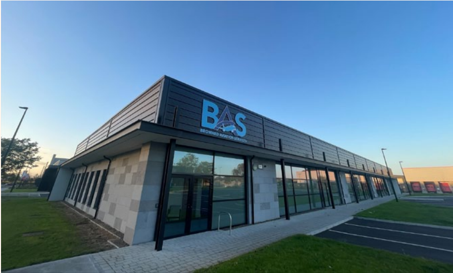
BAS' new facility in Shannon, Ireland
