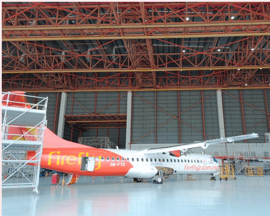
MAB Engineering has doubled its maintenance capacity with the expansion of Hangar 4 at Subang © MAB Engineering
