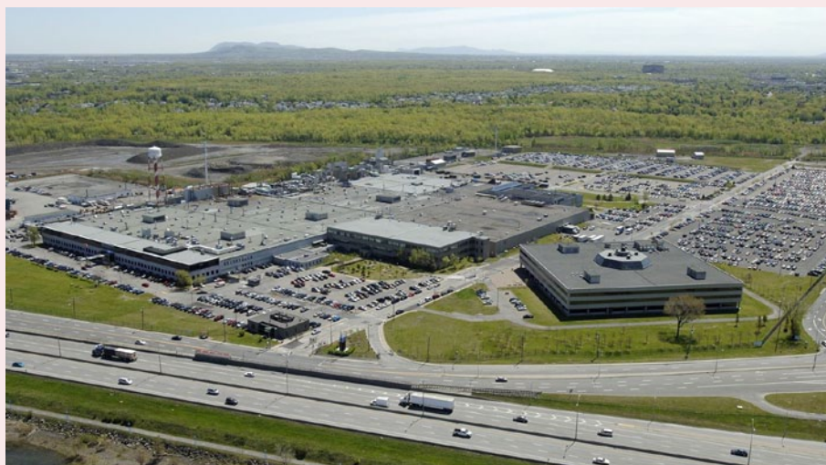
Aerial view of Pratt & Whitney Canada's global headquarters in Longueuil, Quebec
