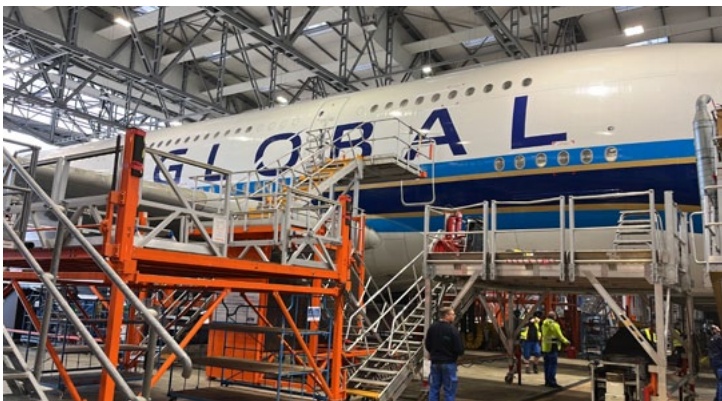
Inside hangar © Global Airlines
