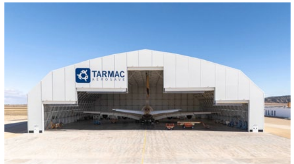
The hangar's innovative design - built with a steel and aluminium frame, and insulated using advanced Rockwool panels - makes it fully dismantlable and reusable © TARMAC Aerosave
