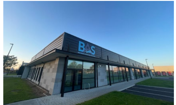
BAS' new facility in Shannon, Ireland
