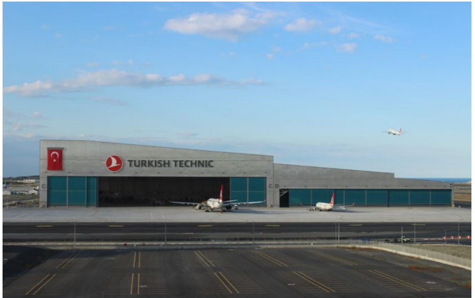
Turkish Technic hangar
