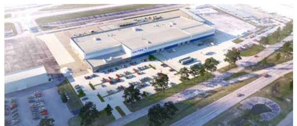
United is breaking ground on a new ground service equipment (GSE) maintenance facility at George Bush Intercontinental Airport (IAH) © United Airlines
