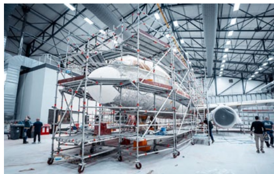
Czech Airlines Technics paint hangar
