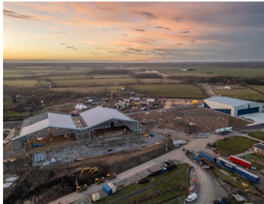
Hangar construction side at Teesside Airport © Teesside International Airport
