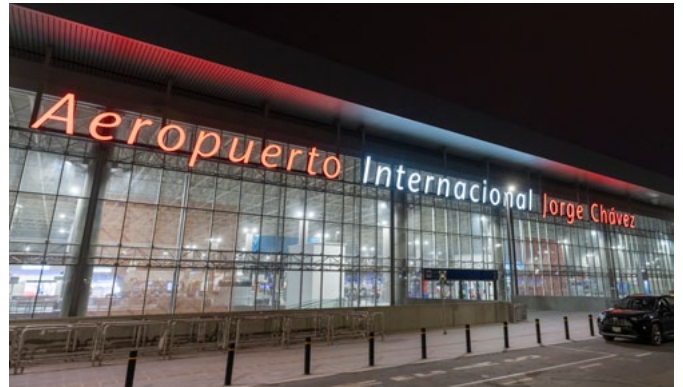
The new passenger terminal at Jorge Chávez International Airport, Lima, has officially opened © Fraport
