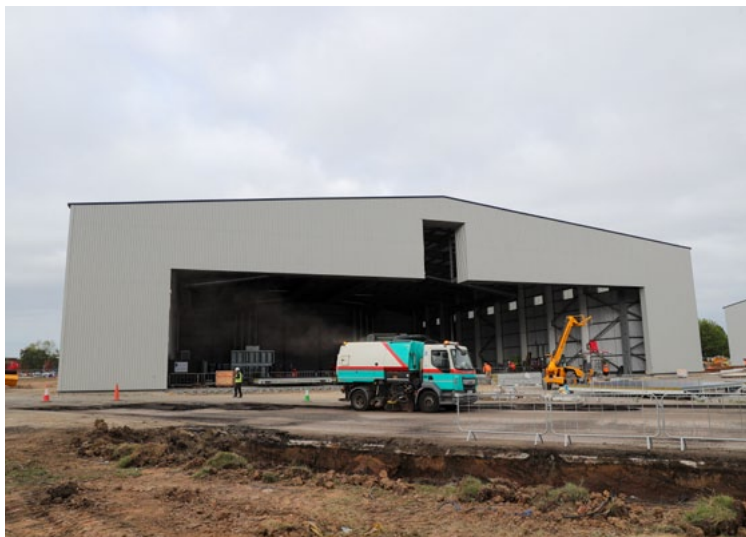
Hangar 9 is nearing completion at Teesside Airport
