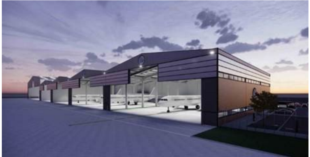
The deal paves the way for the development of up to six new narrow- and wide-body hangars © Teesside International Airport
