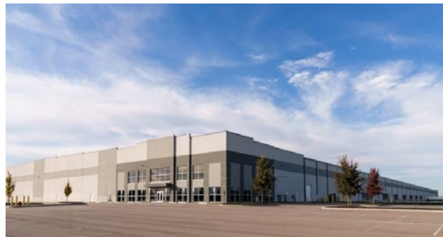
Joby has acquired a new facility in the Dayton, Ohio area
