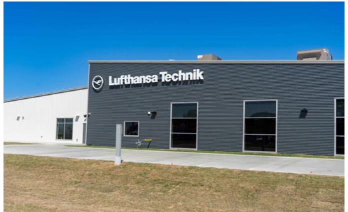
Lufthansa Technik Component Services' new Tulsa facility
