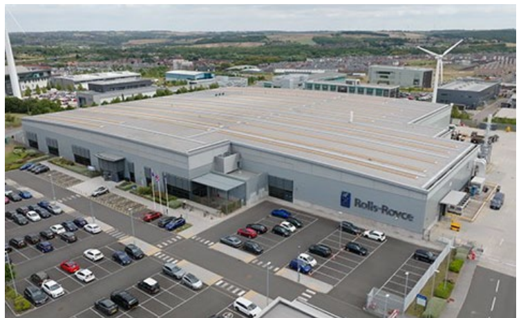
The Advanced Blade Casting Facility, Rotherham, UK
