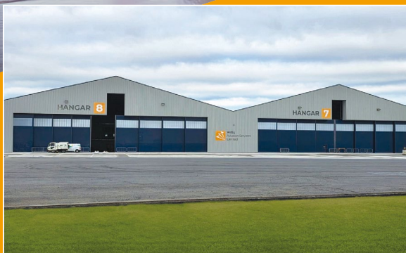
New state-of-the-art twin-bay narrowbody hangars
