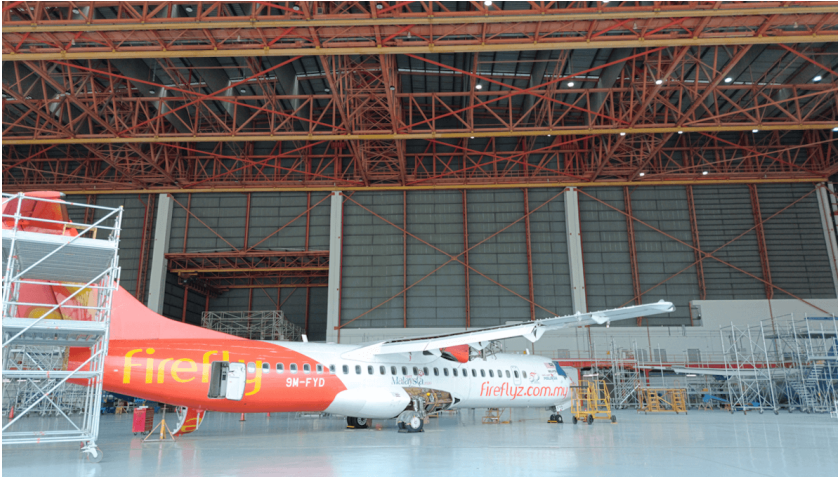
MAB Engineering has doubled its maintenance capacity with the expansion of Hangar 4 at Subang © MAB Engineering
