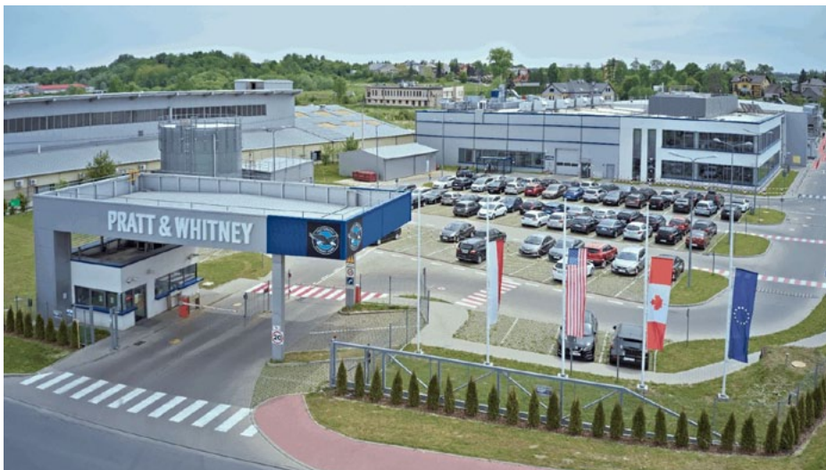
Pratt & Whitney's Niepołomice, Poland, facility
